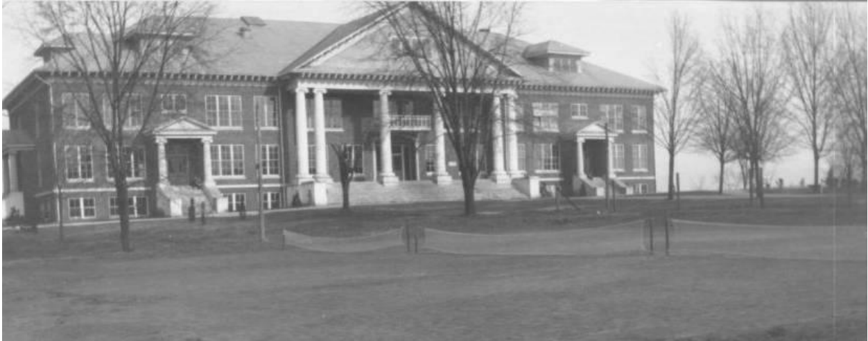
John T. Henderson Memorial Hall Administration Building (Note Tennis Courts on Front Lawn)
